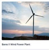
Bares II Wind Power Plant
