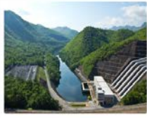
Büyükdüz Hydroelectric Power Plant
