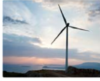
Bares II Wind Power Plant
