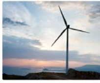
Bares II Wind Power Plant
