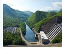
Büyükdüz Hydroelectric Power Plant
